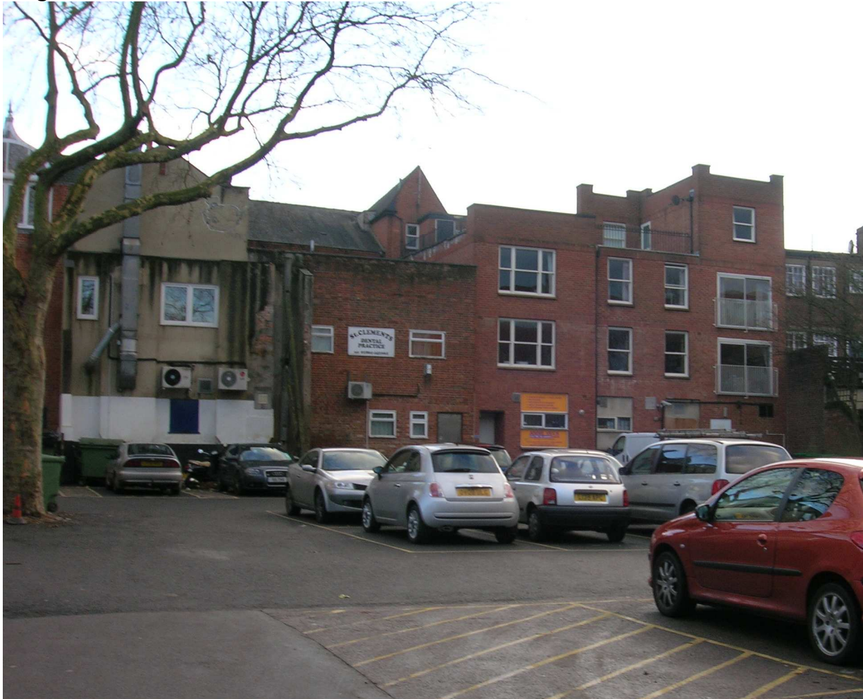
Figure 2: Rear of No 31-38 St Clements
